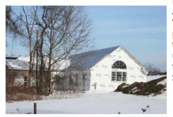
House could not always be accommodated. With a successful fundraising push in spring 2010, we were able to order the timber frame and line up contractors for fall 2010. The foundation was poured in September, the frame was erected in October, and then the rush was on to enclose the building fully before the winter set in. We sighed with relief when during the last week of December, despite frigid weather, the contractor installed the windows and doors to complete that phase of construction.
